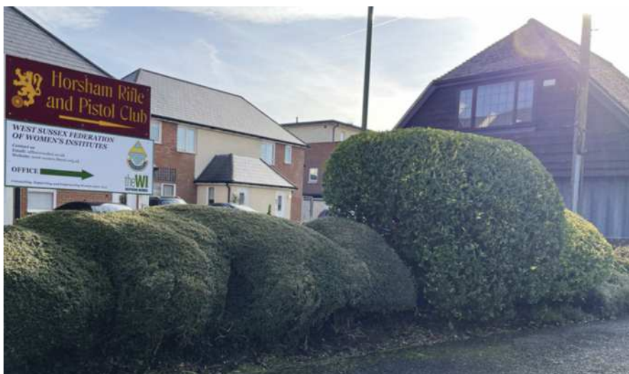
Our new sign and part of our building at Queen Street
